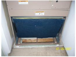
Pull the air filter off from the front of the condenser.
