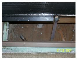
Tygon tubing runs from the drip pan into the drain. Loosen the band clamp with a screwdriver to remove the tubing. Run the tubing under the faucet to clean the inside of the tube. Repeat these steps each year before you start using your air conditioning.
