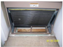
The drip pan is located under the condenser. Remove any water that may have collected in the drip pan.
